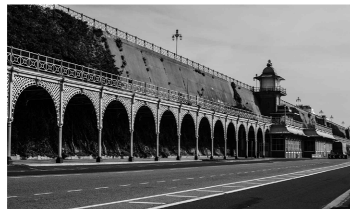
The Victorian iron work before the elements took their toll
